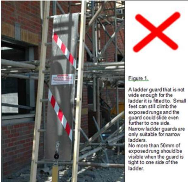
A ladder guard that is not wide enough for the ladder it is fitted to. Small feet can still climb the exposed rungs and the guard could slide even further to one side. Narrow ladder guards are only suitable for narrow ladders. No more than 50mm of exposed rung should be visible when the guard is tight to one side of the ladder.
